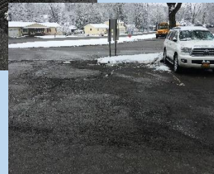
Reconstruct Parking Lots and Sidewalks
