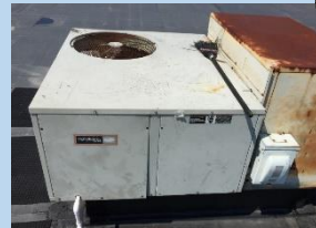
New Heating and Ventilation
